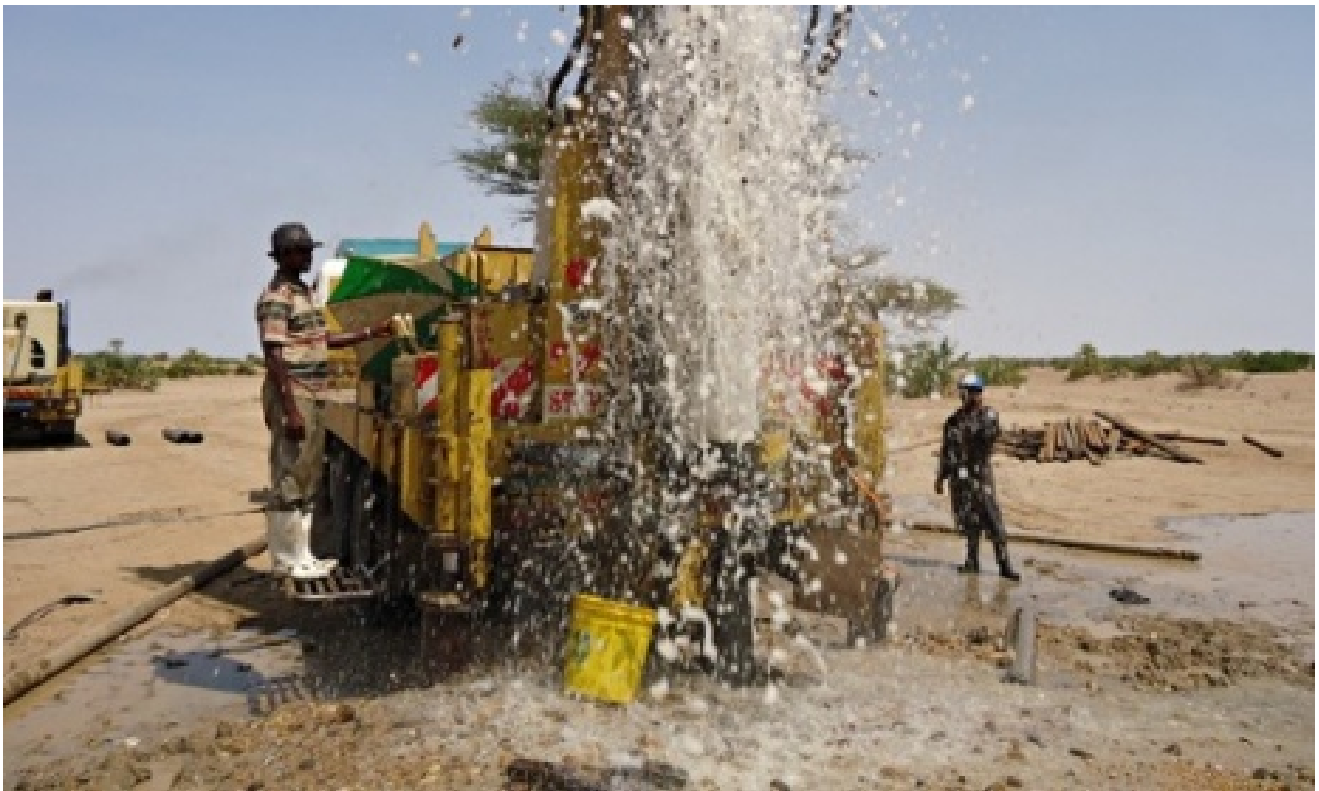
The borehole flushing at Napuu, Lodwar. Photograph: RTI
